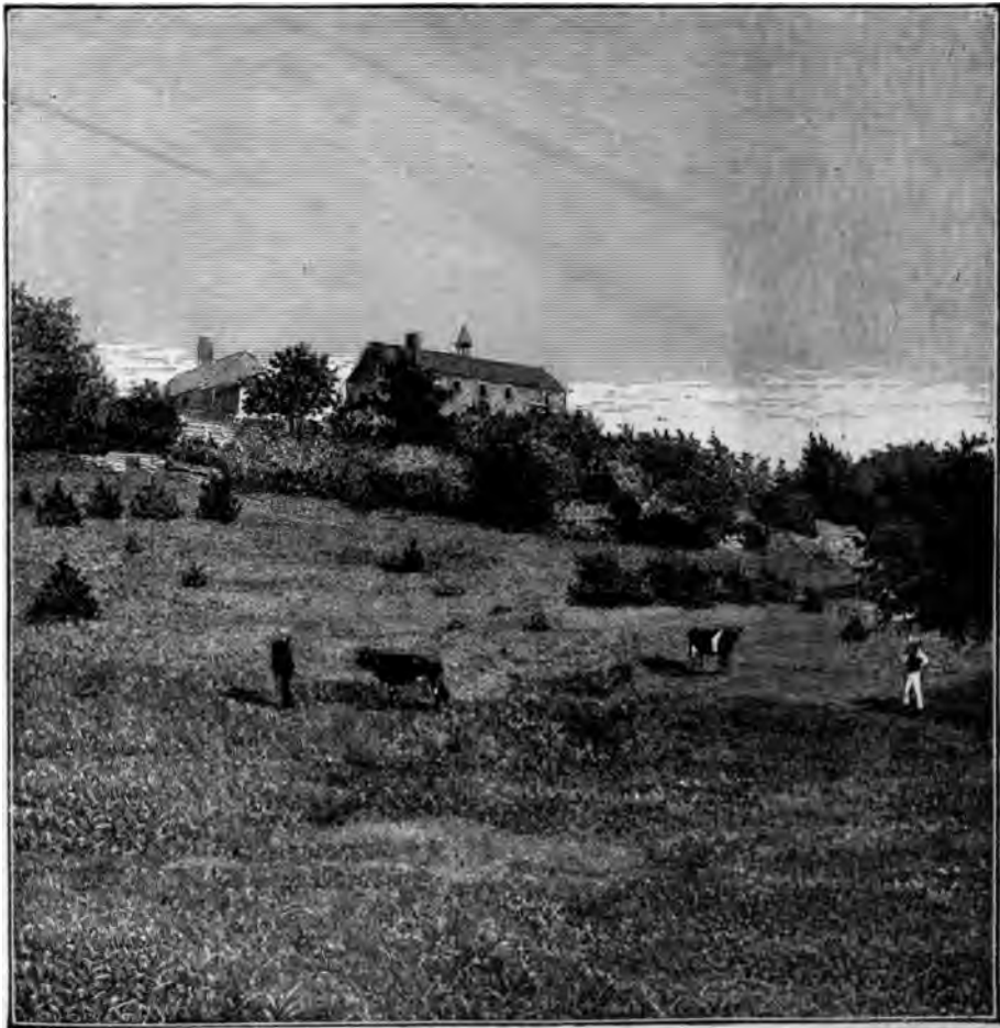
REAR OF THE OLD PRISON, LOOKING UP THE HILL FROM THE WEST. SHOWING KEEPER'S HOUSE AND THE BARRACKS.
